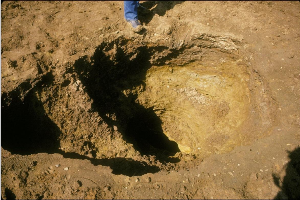
Figure 1. Sinkhole in Garnavillo Lagoon.
